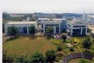
ARAI – FID CHAKAN, PUNE
