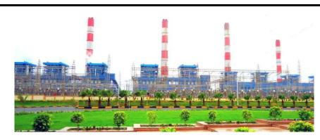
Plant capacity is 4620 MW, comprising of 9 units with 4 units of 330 MW and 5 units
