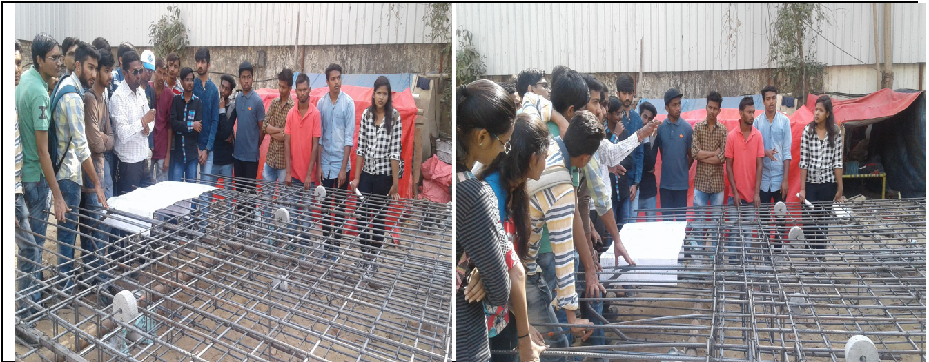
Cage Fabrication with Drawing and Bar Bending Schedule
